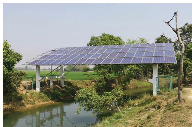
Photovoltaic module over water storage. A photovoltaic module array of a pump system in the Barind region (photo provided by Asian Development Bank consultant).
